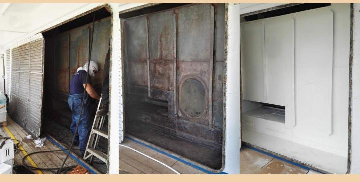
Our turnkey service for external intakes includes: chipping and cleaning the corrupted surfaces, MAD Bond applied to stop corrosion, MAD Fiber applied to restore damaged areas, painting the intakes with MAD Armor.
