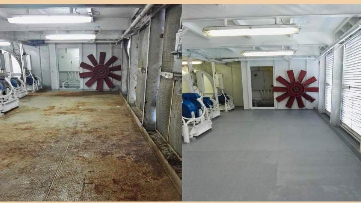
Our turnkey service for external decks and machinery includes: chipping and cleaning the corrupted surfaces, MAD Bond applied to stop corrosion, MAD Fiber applied to restore damaged areas, painting the decks with MAD Shark non-skid, painting of machinery and bulkheads with MAD Armor.
